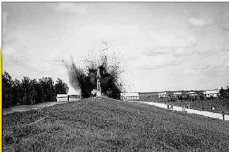
Dynamiting levee south of New Orleans
